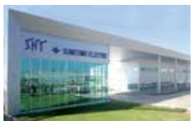
P9 Sumitomo Electric Hardmetal Manufacturing (Thailand), Ltd.
