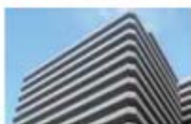
S8 Sumitomo Electric Hardmetal (Thailand) Ltd.
